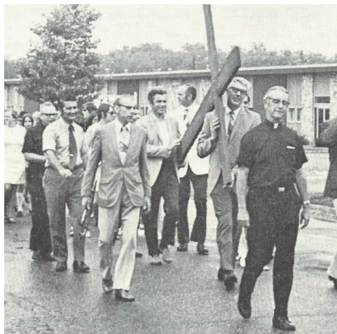
Fr. Kirwin leads the march from the Factory of Love to new property on Kings Highway for the groundbreaking ceremony on Sunday, July 25, 1971
